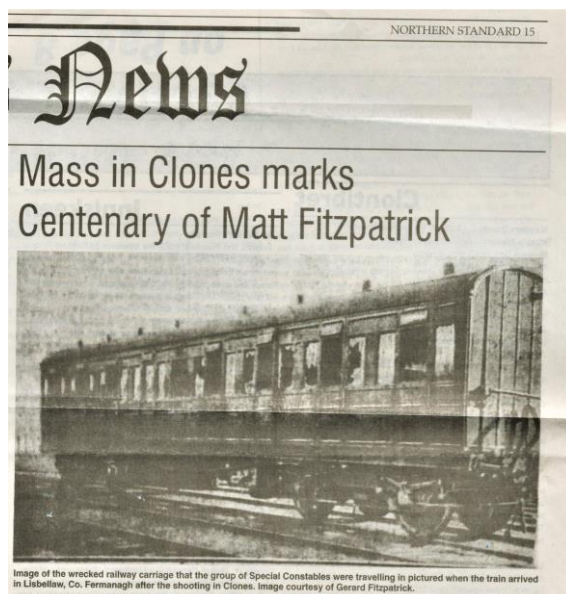
Fig 3: Photo of RUC Rail Car from 11 Feb 2022 Northern Standard newspaper marking 100 years since " Clones Affray ". Photo shows the destruction caused by the Thompson Machine Gun
