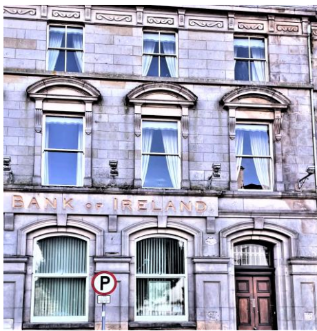
Fig 1: Bank of Ireland Building, Clones. Now an Office complex
